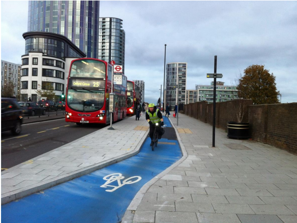
A bus priority lane and bicycle superhighway on High Street, a main arterial leading from Stratford to central London.
